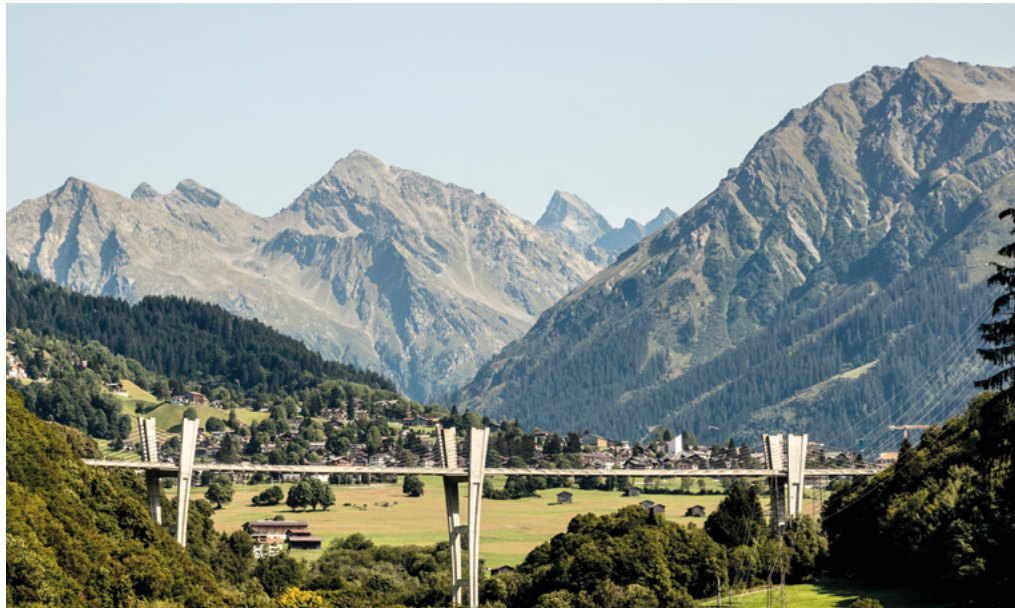
Sunnibergbrücke in Klosters.
